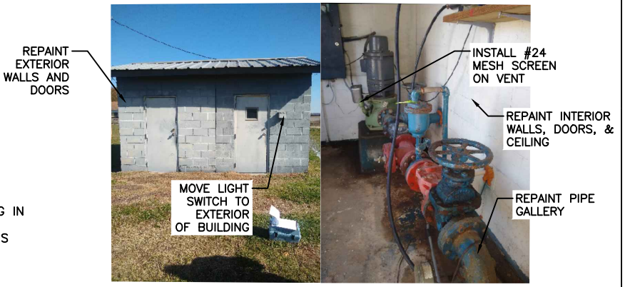
WELL HOUSE NO. 1 REHABILITATION (CONTRACT I)
